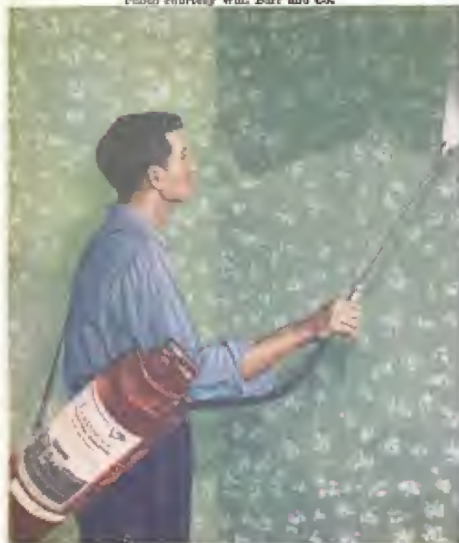
Garden sprayer can be used to apply water or wallpaper-removing solution when taking off old paper. Secret of easy removal is thorough soaking of wall before scraping
